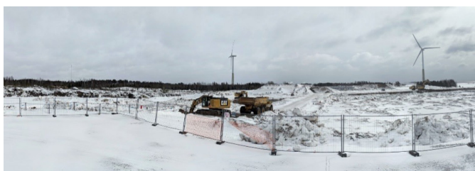
The site before works commenced.
